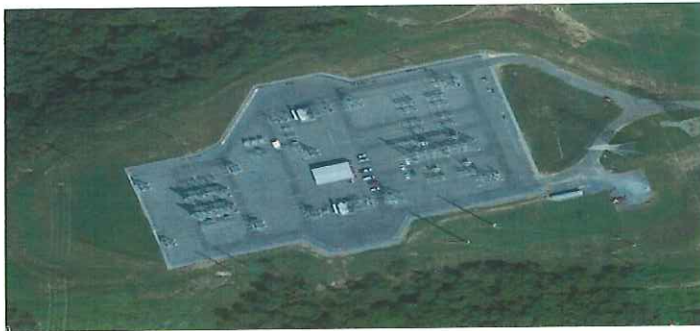
Figure 2: Copperstone 230/69 kV Substation
