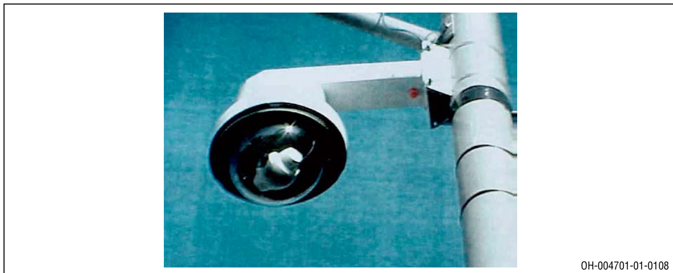
Figure 6.4: Camera Attachment to Metal Pole
