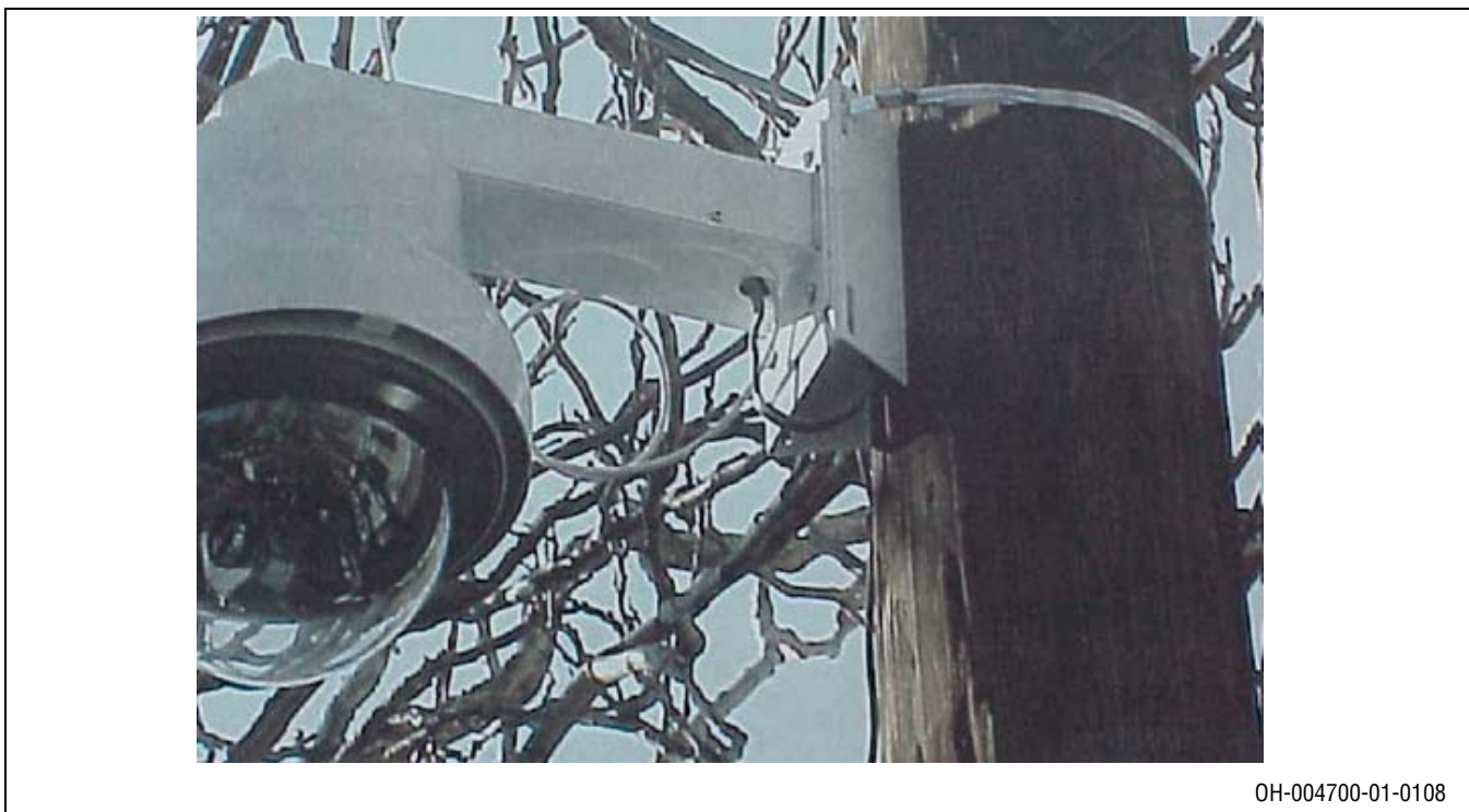
Figure 6.3: Camera Attachment to Wood Pole
