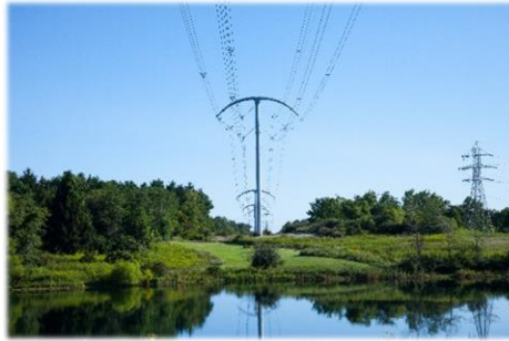
345kV BOLD Double-circuit (3-conductor)
