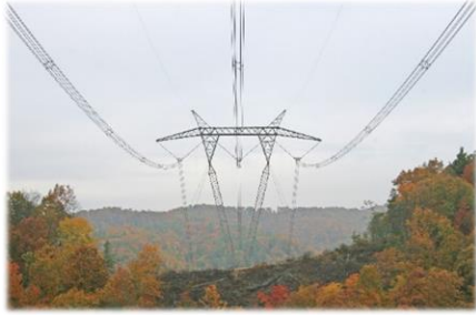
765kV Single-circuit (6-conductor)
