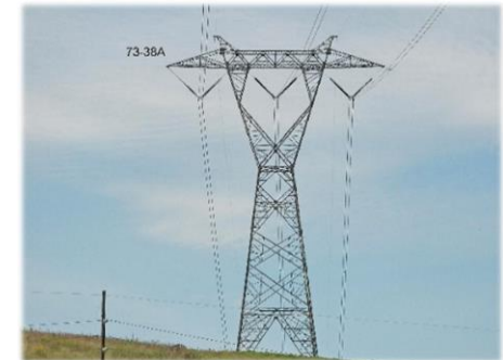
500kV Single-circuit (3-conductor)
